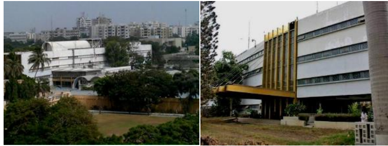
Figure 1: U.S. Embassy, Karachi Pakistan with slit windows running on façade. Photos by © Architect Arif Bilgaumi, used with his permission.
