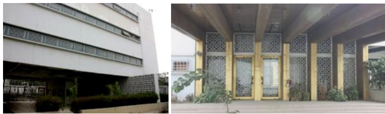
Figure 4: Perforated wall and Geometric Screens used in U.S. Embassy Karachi. Photo by © Ar Arif Bilgaumi, used with his permission.
